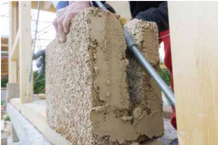
Detail of CANAPLOCK with wooden frame.
